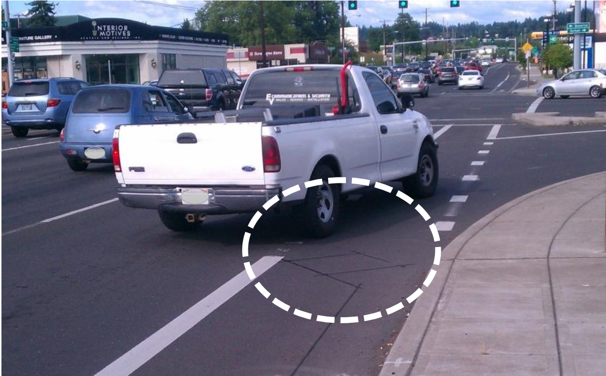
1 2 FIGURE 8 OR-99W eastbound approach towards Portland 3 Note: See location of inductive loop relative to right turning vehicle – within dashed oval
