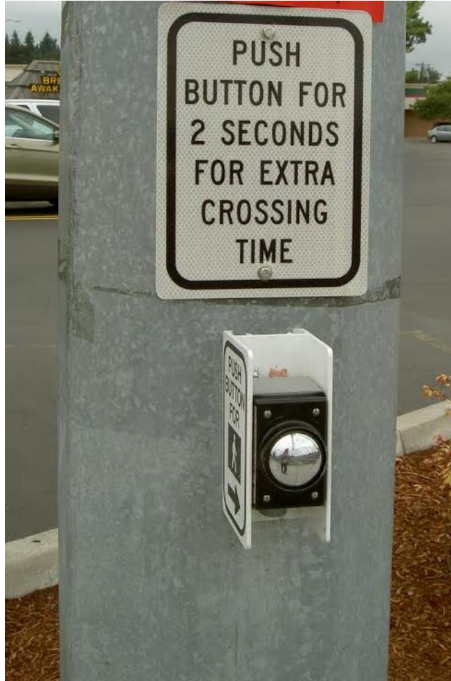
1 2 FIGURE 2: Pedestrian Phase Actuation Button (NW Quadrant of Intersection of OR-99W and Hall 3 Boulevard, Tigard, OR)
