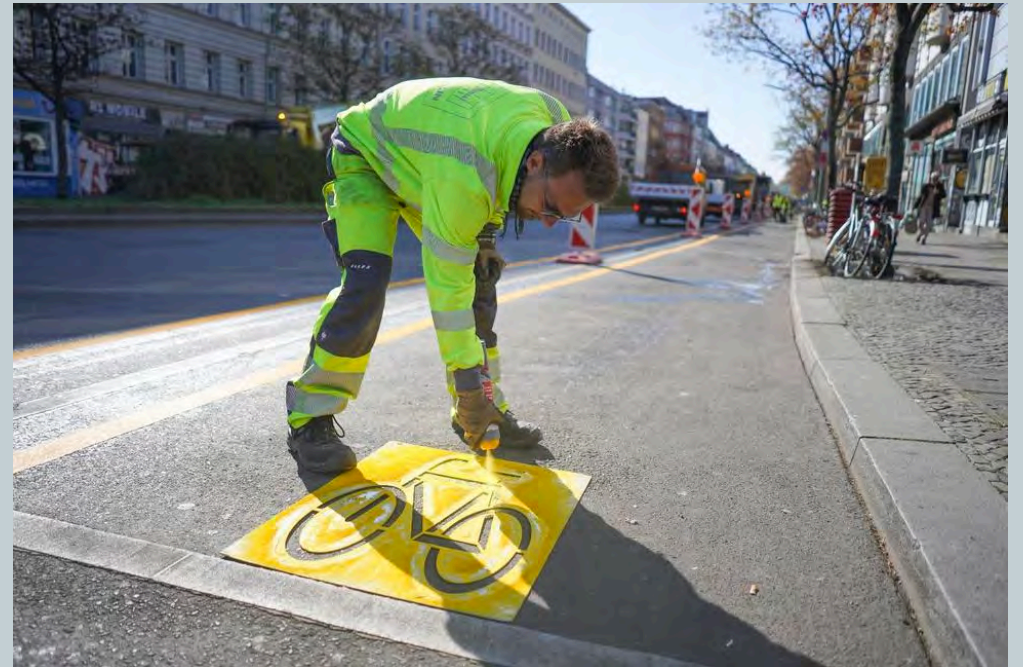
Painting a temporary bike lane in Berlin, Germany
