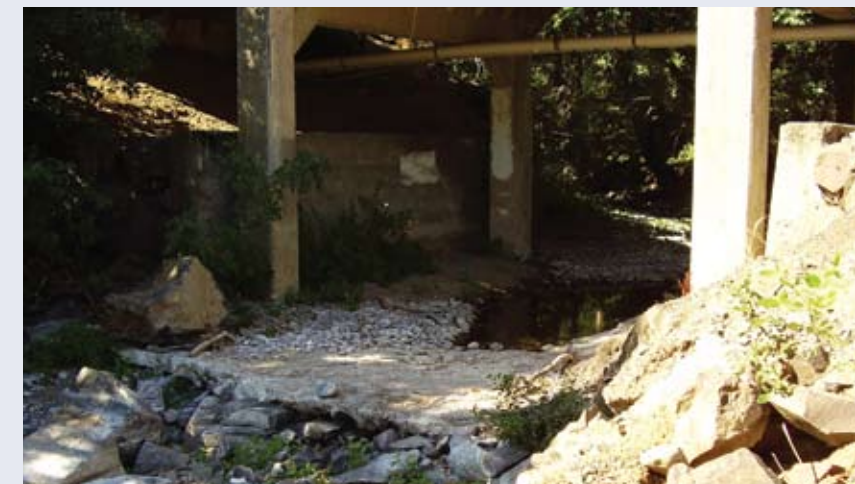
Example of a roughed chute failure where channel bed scouring and loss of above-ground water flow prevent fish passage (Chenoweth Creek, OR). Photo courtesy of Hamid Moradkhani.
