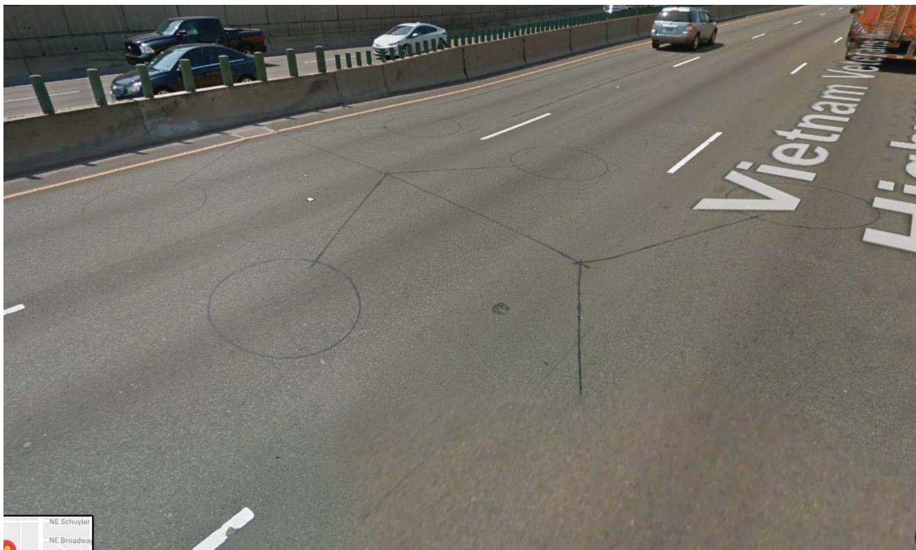
Figure 1-4: Google Streetview (Google, 2019) at WB I-84 Halsey Ramp, MP 5.82 (ID's: 101159-101161)
